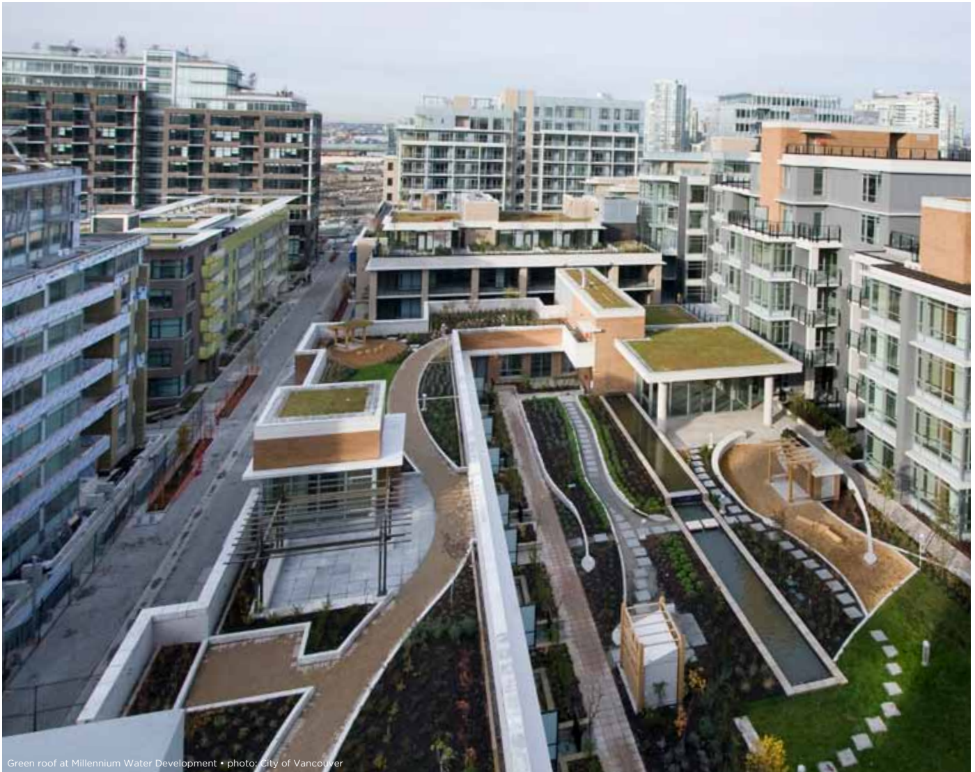
Green roof at Millennium Water Development • photo: City of Vancouver
